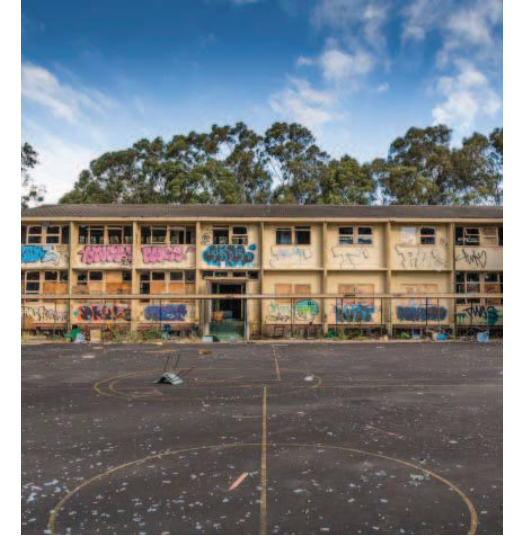
THE FORMER MACQUARIE BOYS HIGH SCHOOL
