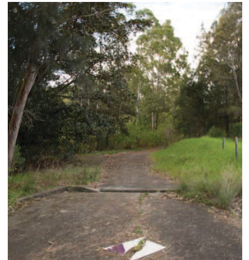
FORMER ONE LANE ACCESS ROAD TO SCHOOL
